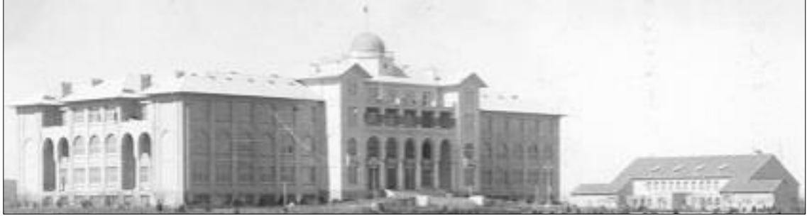
Fig. 131: Front view of the Gazi Education Institute and the Department of Physical Education buildings on the right, captured in 1932. Source: Dr. Niyazi Altunya Archive
