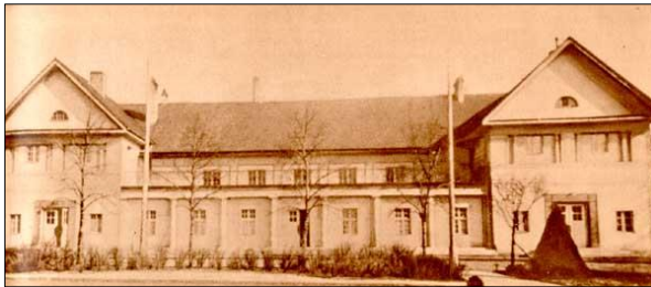
Fig. 153: The building of the Department of School Hygiene and Physical Education, Wilson Park, Poznań, 1921. Source: https://awf.poznan.pl/uczelnia/o-nas/ Academic authorship: prof. dr hab. Maciej Łuczak
